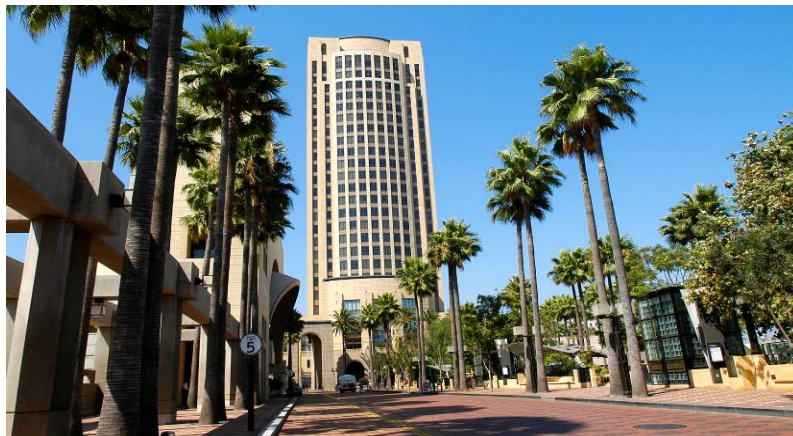
Patsaouras Transit Center and Metro's Gateway Headquarters in downtown Los Angeles
